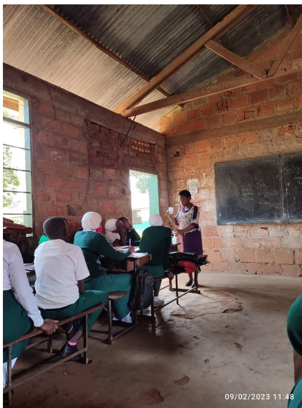
Figure 4.12: A chemistry lesson at MSS conducted in the classroom due to insufficient space in the school science laboratory. (Field, 2023)
